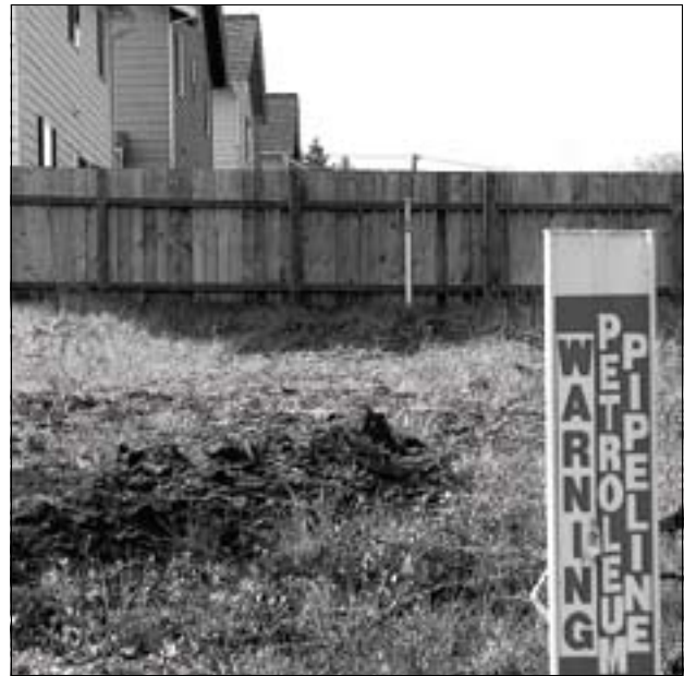
A hazardous liquid pipeline running 15 feet from people's backdoors.
