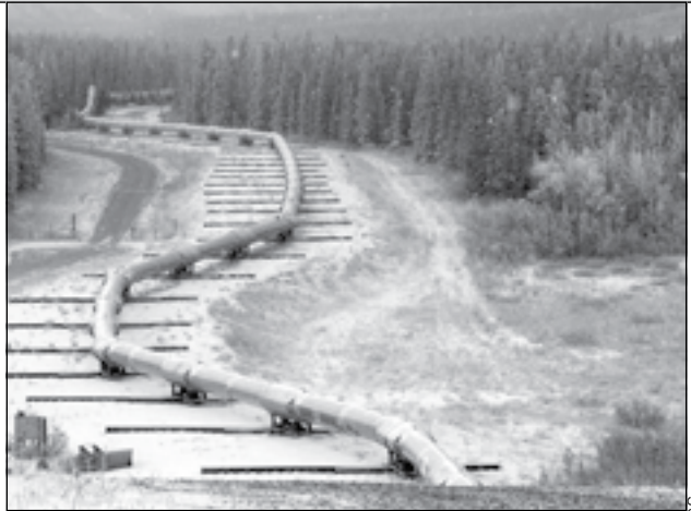
A part of the Trans-Alaska Pipeline, near the Denali Fault, designed to withstand earthquake movements.
